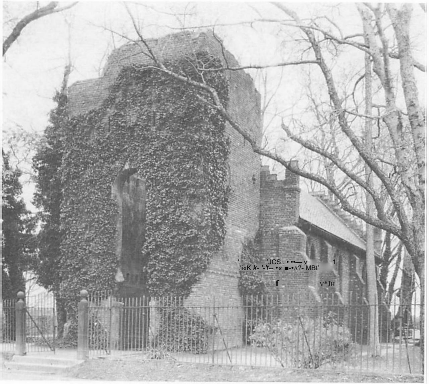
OLD CHURCH TOWER
